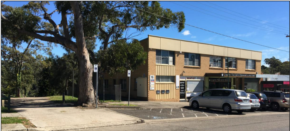
Figure 4 – Neighbourhood Shops on northern boundary of Site adjacent Taylor Avenue
